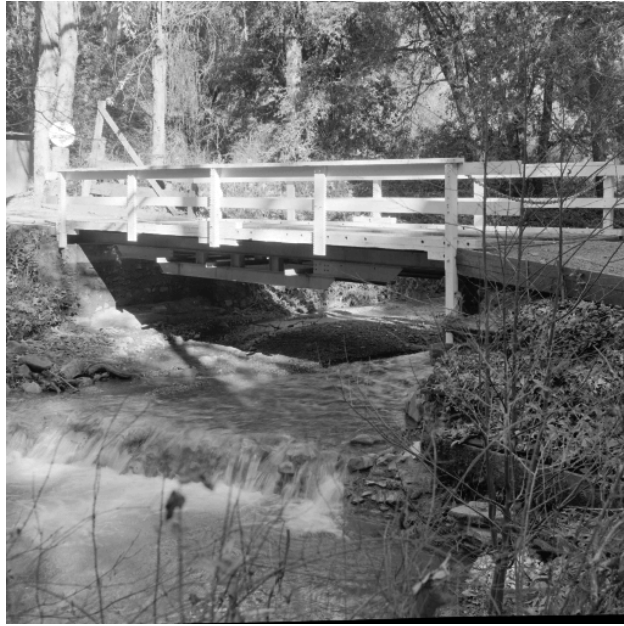
Fig. A.8. Bridge: original image
